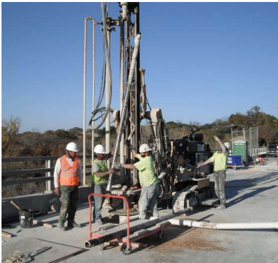
Figure 8. Drilling Rig on Left Abutment
