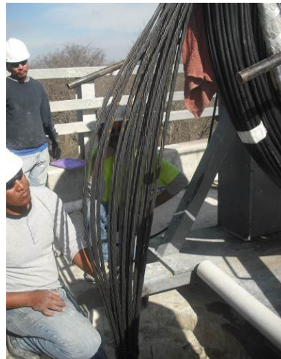
Figure 19. Strand Tendon Opening up During Uncoiling
