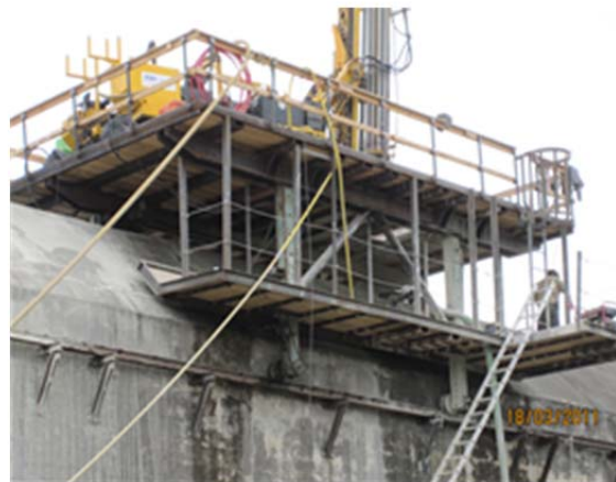
Figure 11. Moving Platform at Overflow
