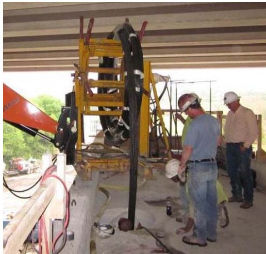
Figure 18. Installing Tendon with Uncoiler under the bridge
