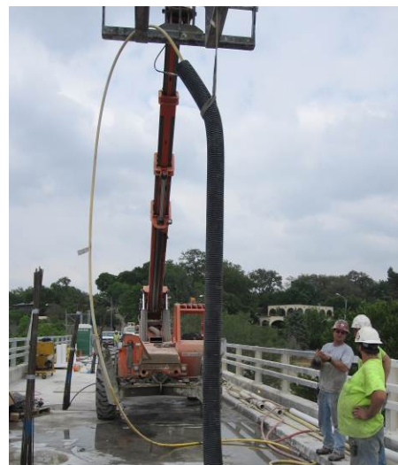
Figure 17. Corrugated 12 feet above grade for Leak Test
