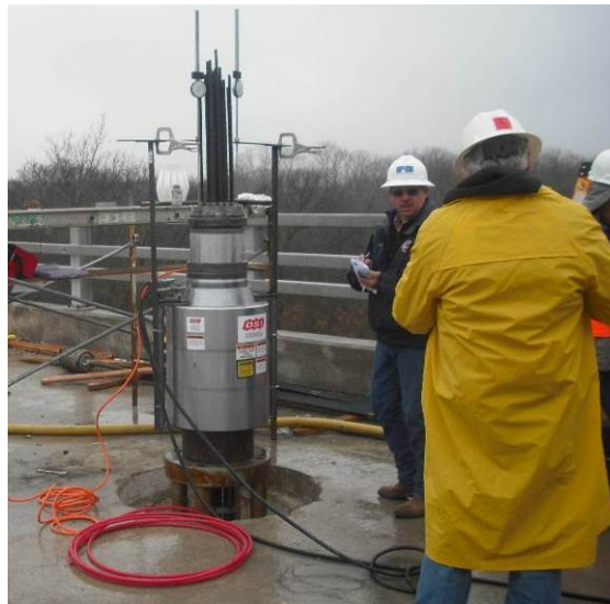
Figure 20. Performance Testing a 20 Strand Tendon
