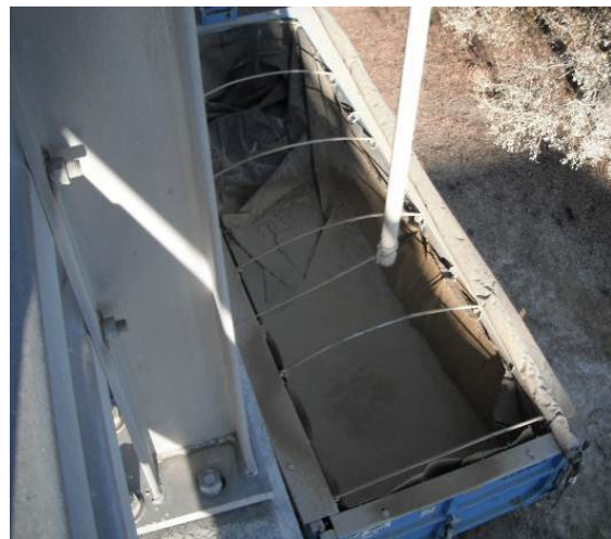
Figure 15. Steel Roll Off Tank for Cut Drilling Waste
