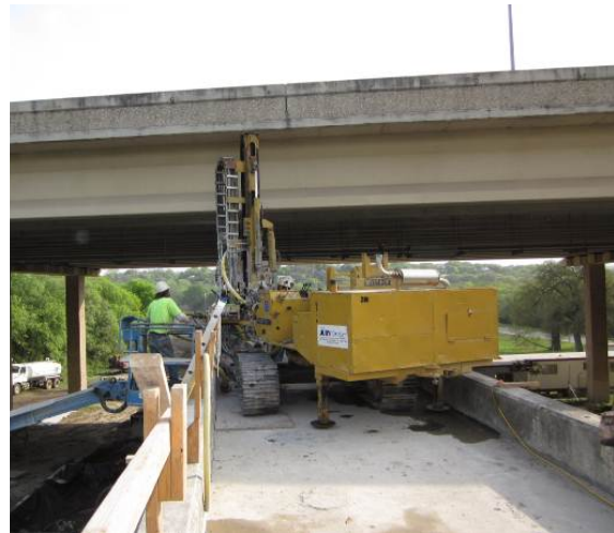
Figure 13. Rig at Right Non-overflow Section
