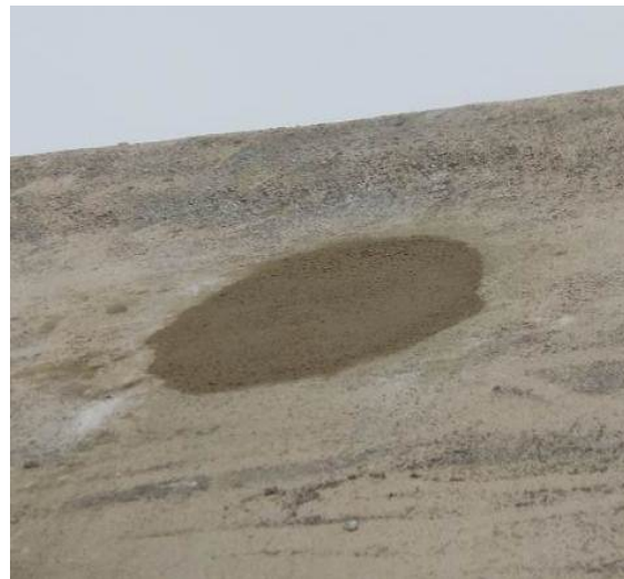
Figure 22. Lean Concrete Backfill on Ogee Anchor Holes
