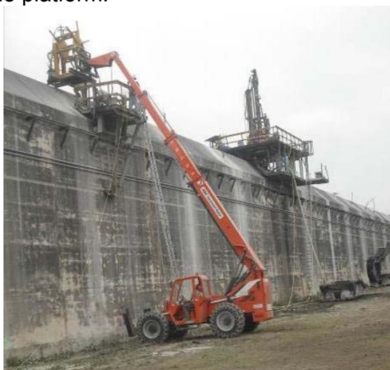
Figure 10. Access to Overflow Section
