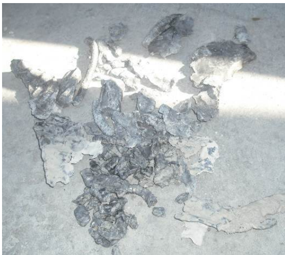
Figure 14. Steel Removed from One Hole
