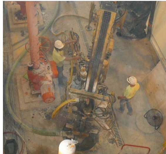
Figure 9. Limited Access Drill in Gatehouse
