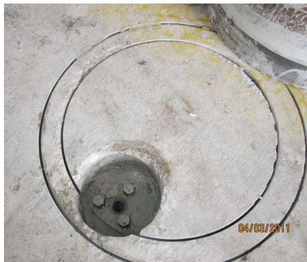
Figure 6. Pocket Overlap with Existing Anchors
